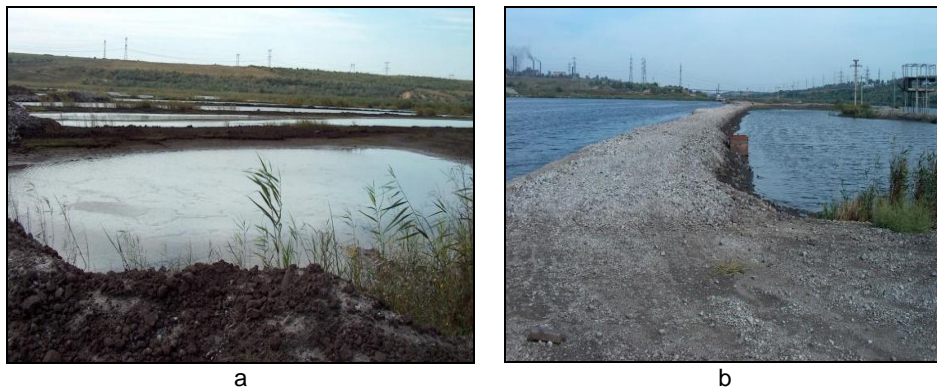
Fig. 2 Ponds for liquid and industrial wastewater decantation: a - general view of the pond with the settling basins; b - detail of the pond partition.
